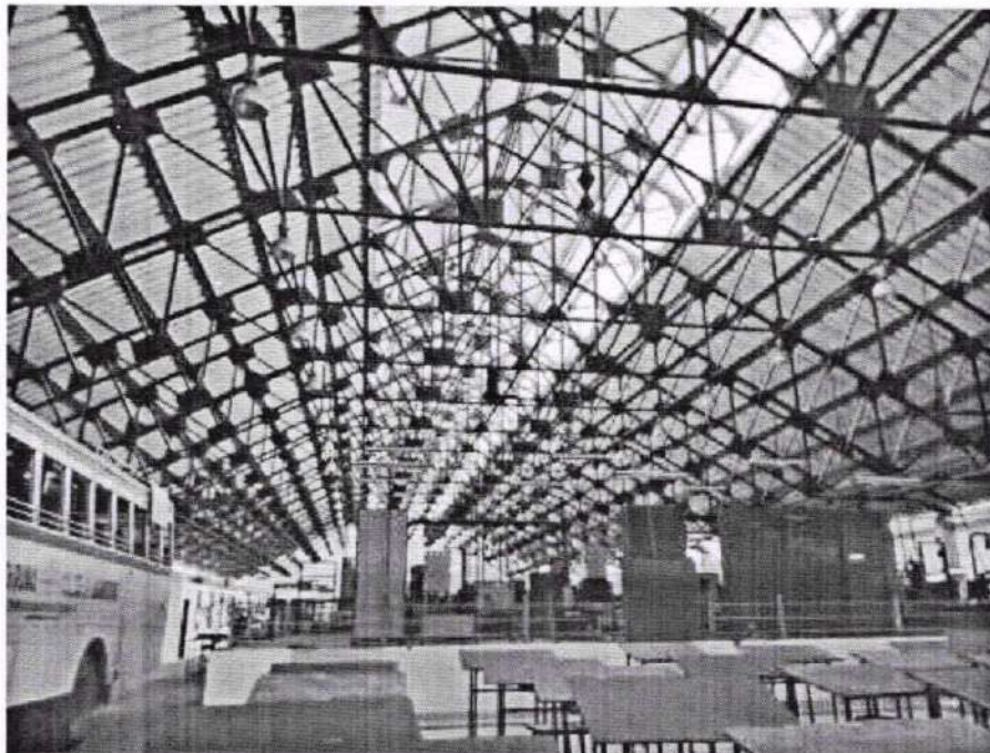
Figure 8: Lack of heat exhaust systems in lab building
